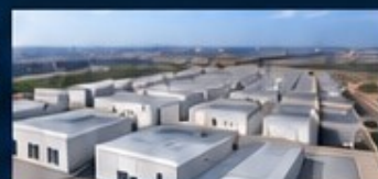
LUXOR INDUSTRIAL CITY Industrial MEP Works
