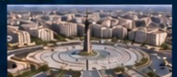
PEOPLE'S SQUARE Urban Development MEP Works
