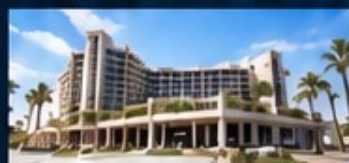
TOLIP ALAMEIN HOTEL Hospitality MEP Works
