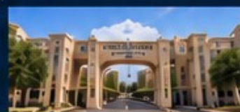
ZAGAZIG UNIVERSITY Educational MEP Works
