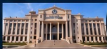
SENATE New Administrative Capital Governmental MEP Works
